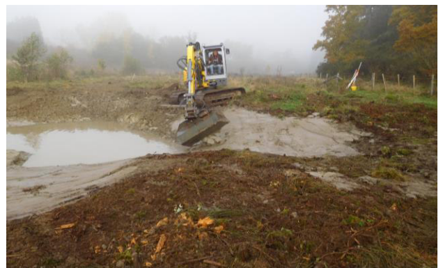
Two ponds were dug to excavate soil to fill up the ditches.
