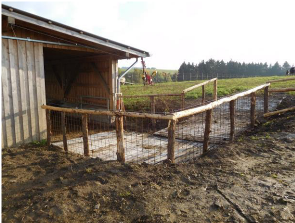
Installation of boards at the entrance of the shelter to prevent the erosion of the soil due to the trampling of the Galloways.
