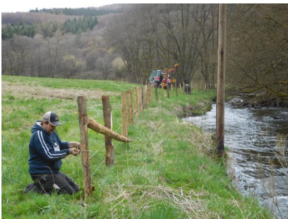
Attaching of wire to the posts by CNDs at the site Schleef.
