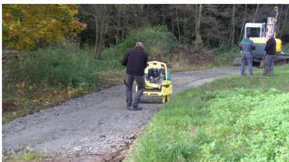
Rolling of the gravel for reinforcement.
