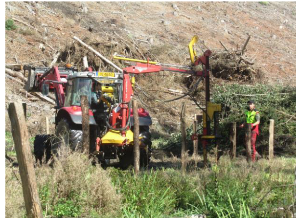
Installation of posts for the construction of a fence in Breitwies by CNDs:
