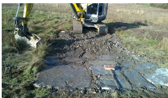
The new ford with large stones is a durable solution.
