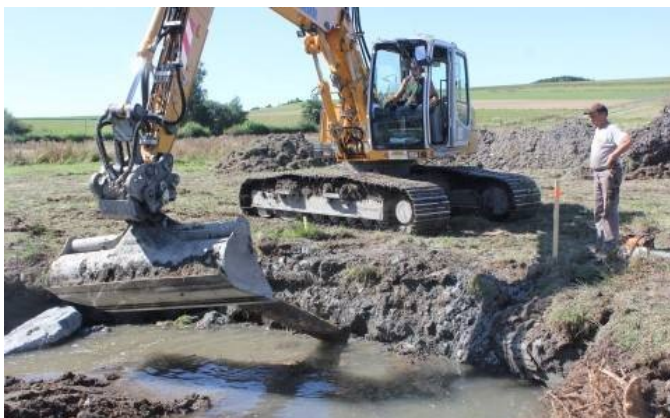
Tree stumps were introduced into the riverbank to diversify available habitats in the new course of the stream.
