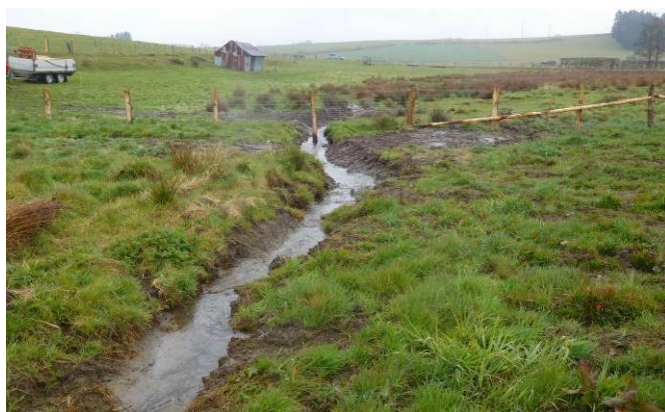
The stream Fennbaach was relocated into its thalweg.
