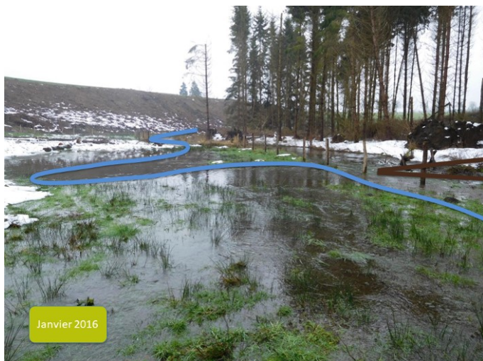
The deflector (in brown) at Breitwies successfully deviated the Tretterbaach (in blue). Unfortunately it was washed away during the winter 2016.
