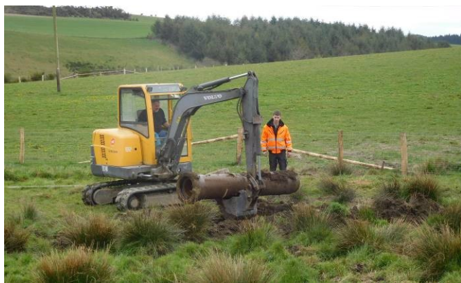
Several drainage pipes were removed at Fennbaach .
