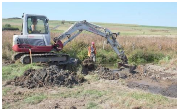
The last step of the remeandration project was the dredging of the plug separating old and new riverbed.
