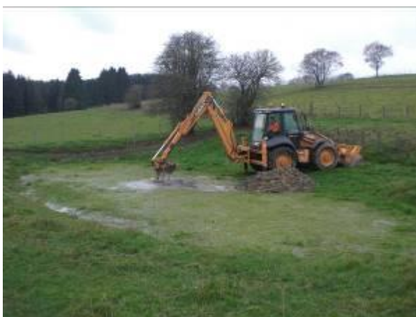
Figure 35. Excavation of sedimented pond in Kaleburn (19.07.14)
